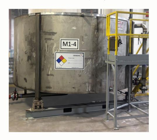
M1-4 Tank Equipped with shotgun lines, load cells, VFD, and 350' of 2" spiral heat exchange coils
